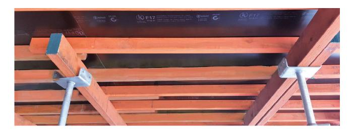
Laminated veneer lumber is intended for use on concrete formwork, joists, bearers, walers, soldiers and supports It is strong, lightweight, straight and uniform which will reduce forming costs and improve the quality of concrete finish.
